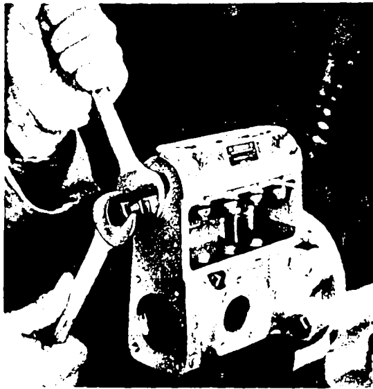
Fig. 36 Unscrew control-rod guide bush with extractor
